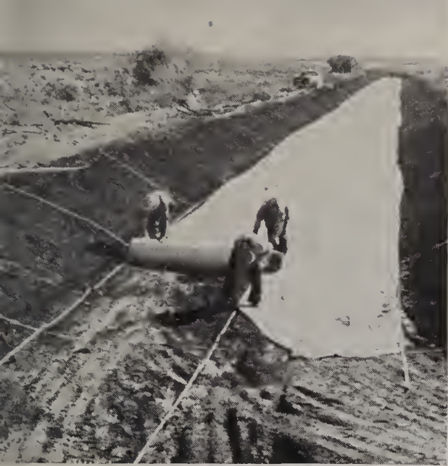
Cotton linings are used in building ditches and canals in arid sections.
